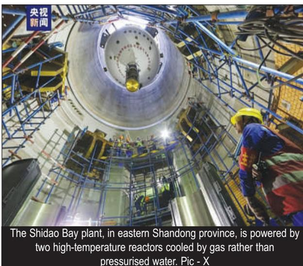
The Shidao Bay plant, in eastern Shandong province, is powered by two high-temperature reactors cooled by gas rather than pressurised water. Pic - X
